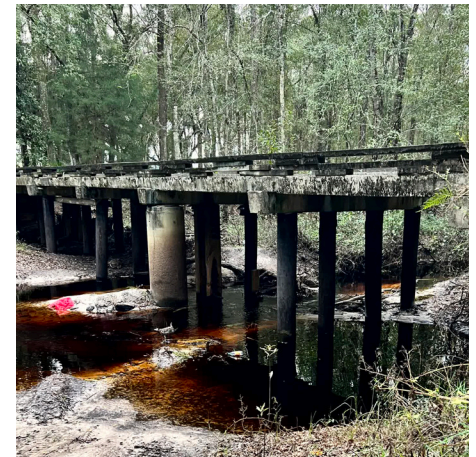
Richardson Road Bridge
