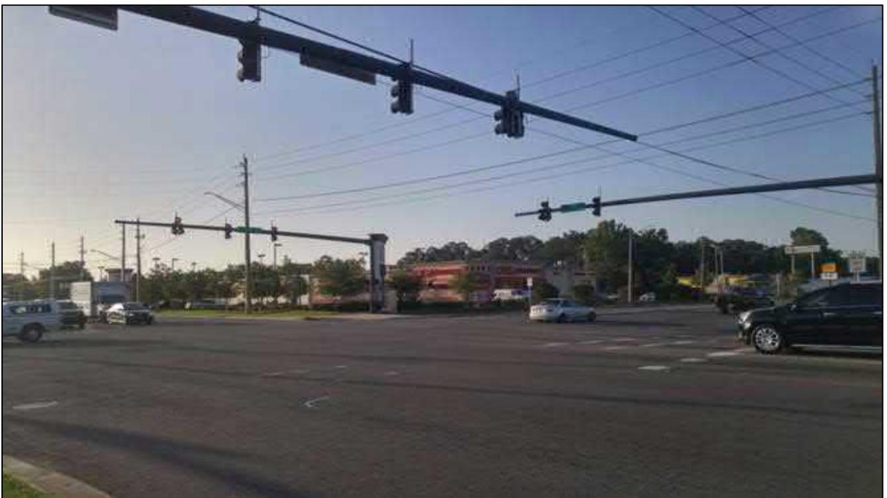
Photo 2: Looking southeast – Faded crosswalk on the west leg
