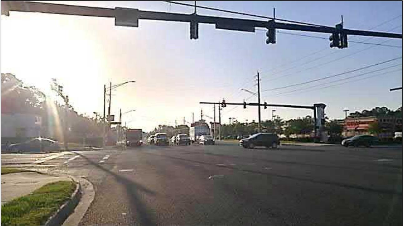
Photo 1: Looking East – Sun Glare (no backplates for the signal heads)
