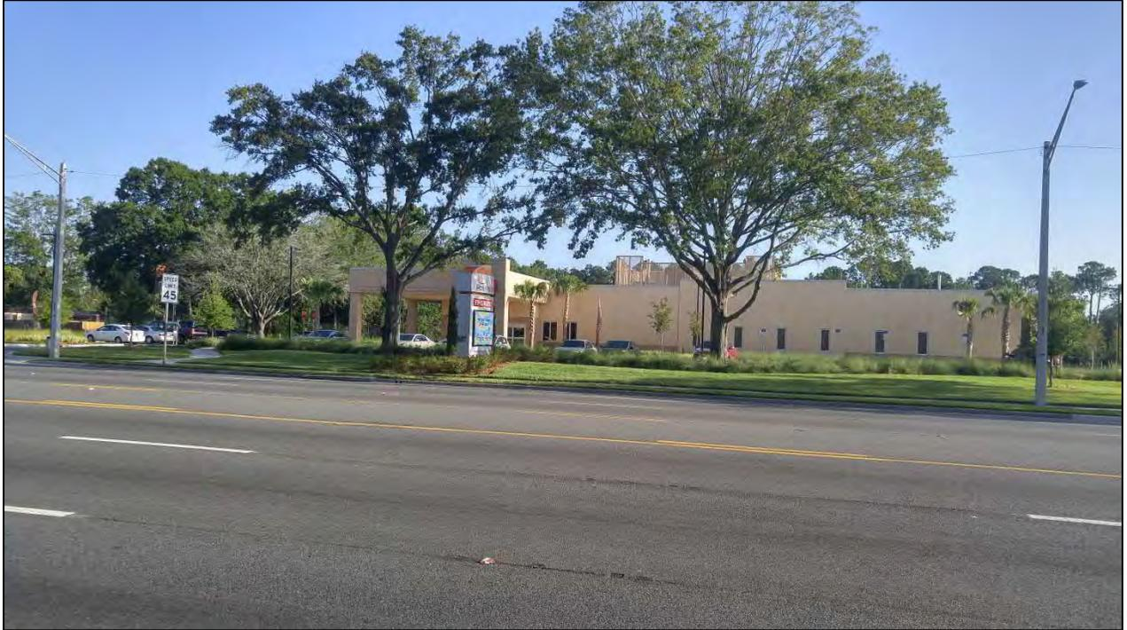
**Photo 3: South leg: Note faded pavement markings 125 feet south of the intersection**
