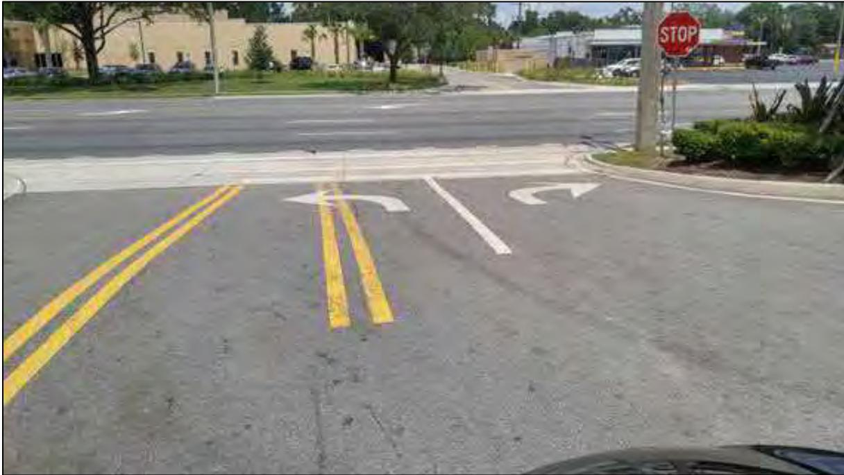
**Photo 5: Looking north: Note improper pavement marking at Dollar Tree driveway**
