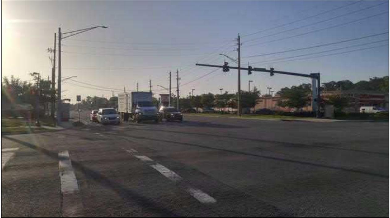
**Photo 3: Looking East – Faded crosswalk north leg and pavement rutting**
