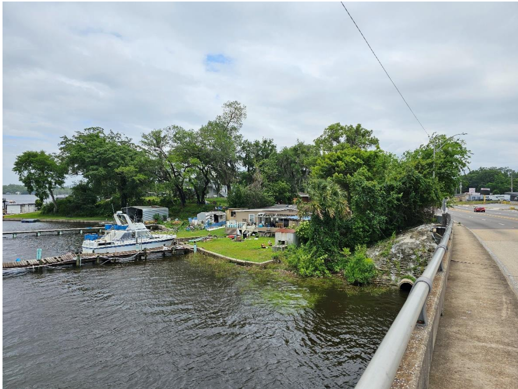
2) Looking southeast from the existing Lem Turner Road bridge over the Trout River at Proposed Pond Site 1.
