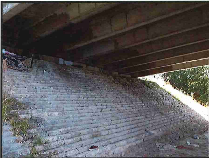
Project No: 631017420 Photographer: William Zukauskas Description: Bridge #720033 abutment.
