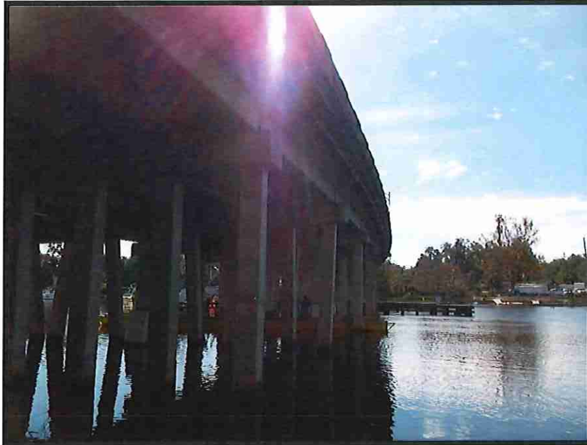
Project No: 631017420 Photographer: William Zukauskas Description: Bridge #720033, facing north
