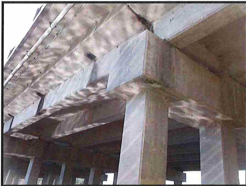
Project No: 631017420 Photographer: William Zukauskas Description: Bridge #720033 support and deck drains
